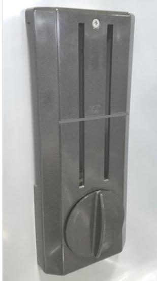
**Spa Skimmer:** This device is located at the water level of the spa. It pulls debris from the surface, pre-filters the water through the "Skimmer Basket", and then pumps the water through the fiber filter. The Skimmer Basket should be cleaned about once every two (2) to four (4) weeks. The basket is removed for cleaning by un-threading the Skimmer Retainer and removing the basket. There is a "Water Level" line on the Skimmer to help you maintain the right water level for your spa.
